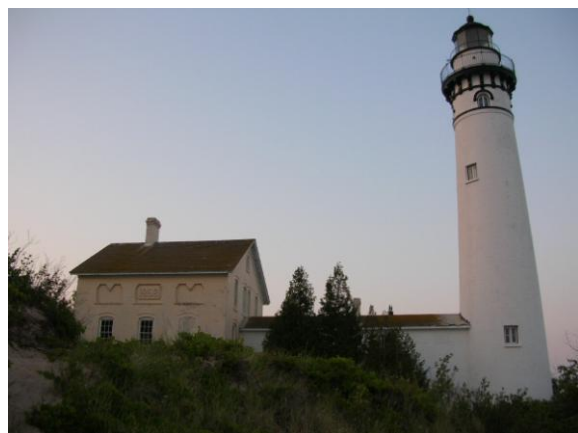
Keeper's Quarters, walkway to lighthouse and 1871 Lighthouse tower.
