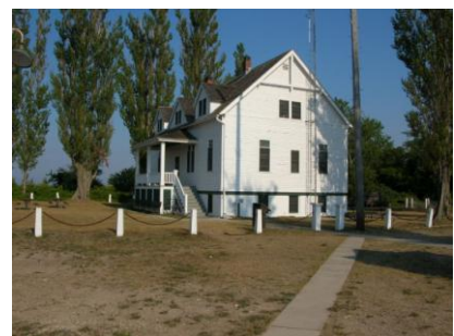
SMI USLSS and NPS Ranger Station 2007
