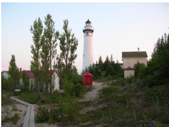
Lighthouse complex – Fog Signal building on left, small cylindrical building in the center is the flammable storage building.
